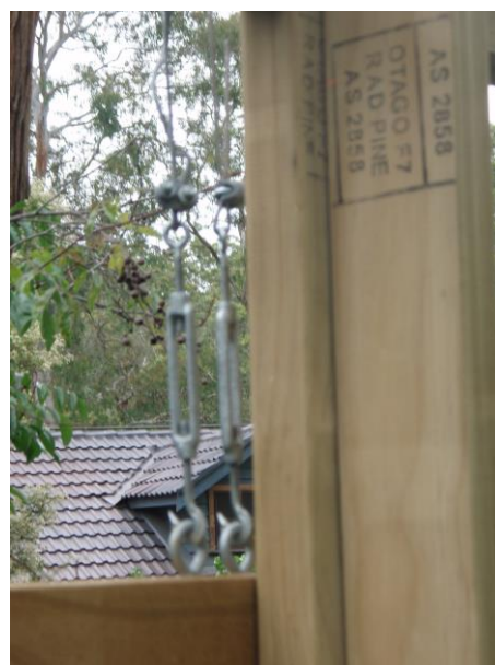
Figure 4: Tensioning devices for the cables
